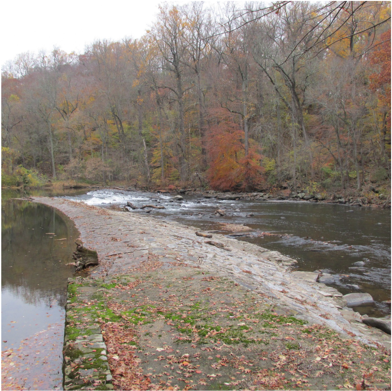
Dam 9 Looking Upstream East Bank, Partially Breeched
