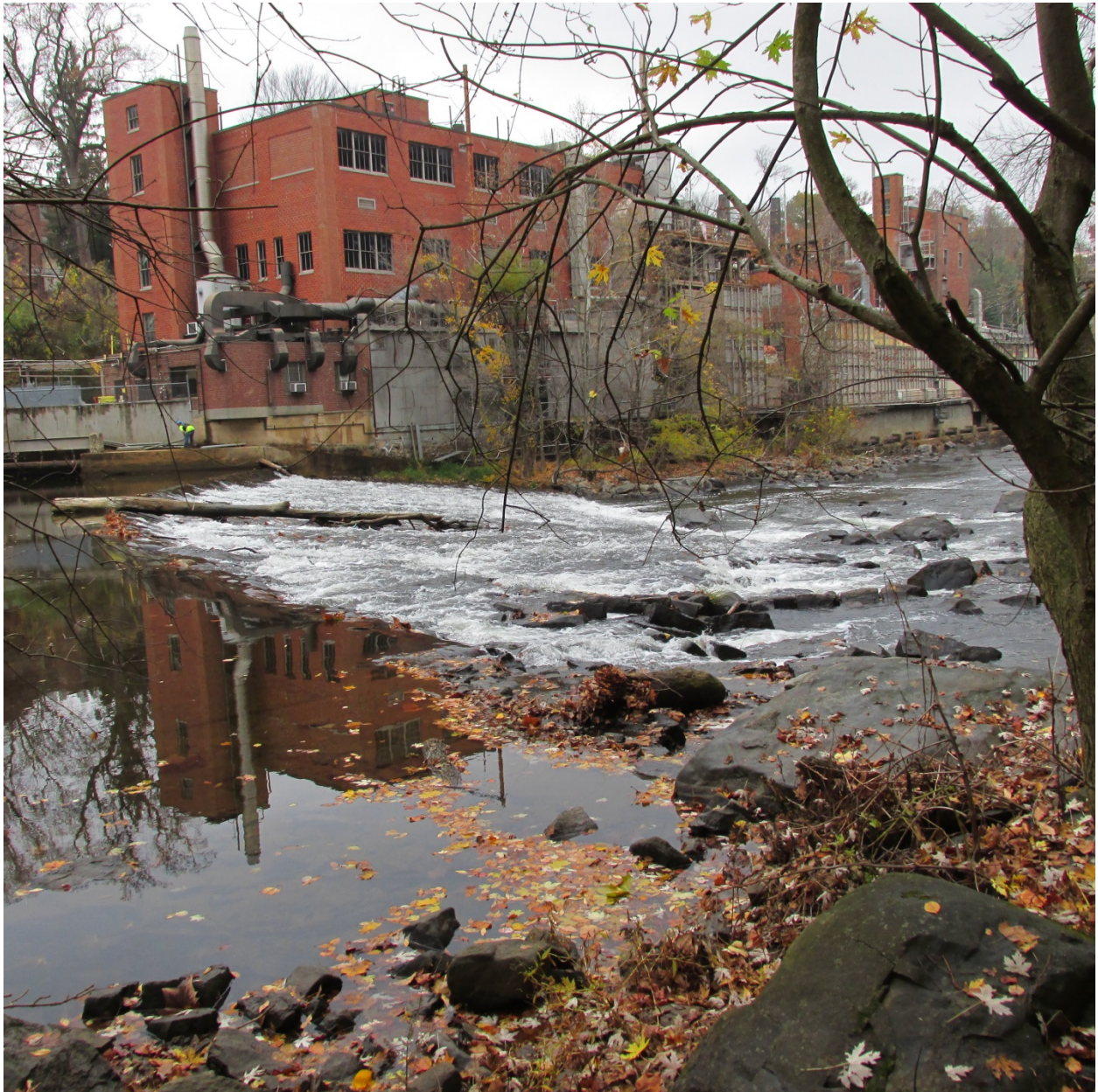
Dam 6 Looking Downstream, Partially Breeched
