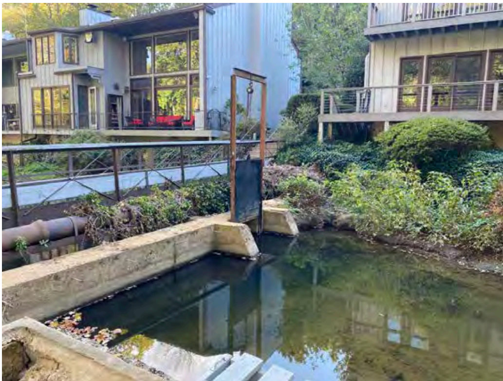
Plate 6.8: Overview of a smaller sluice gate along the millrace, further controlling the water flow to the former Bancroft and Sons Cotton Mills complex.
