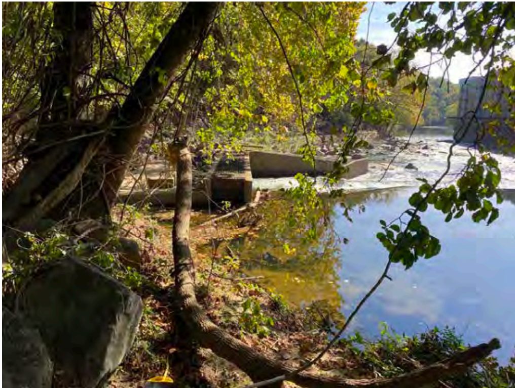
Plate 5.7: Overview of an abandoned concrete technical fishway and a concrete encased sewer line on the north side of Dam 4.
