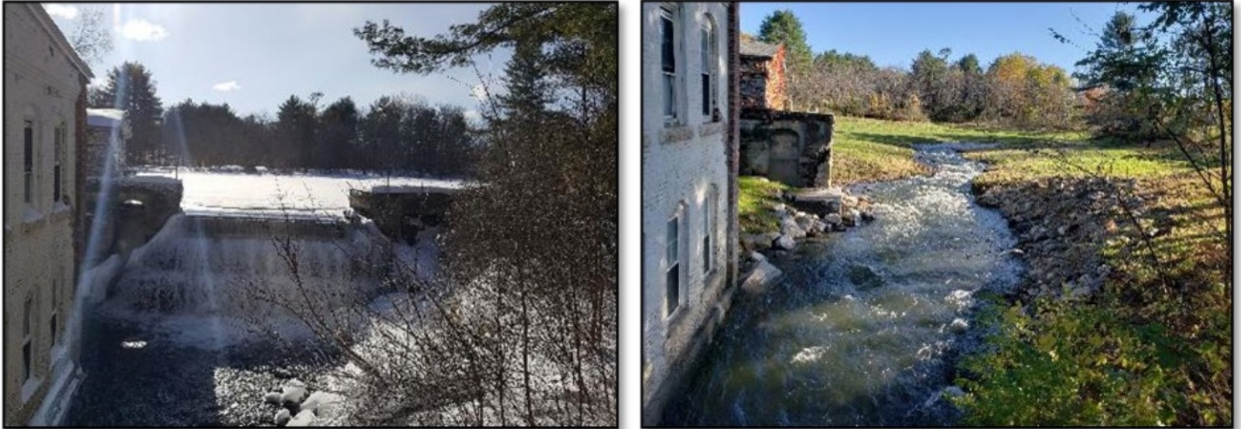
Figure 4. Example Partial Dam Removal by Kleinschmidt - Lombard Dam; Vassalboro, Maine
