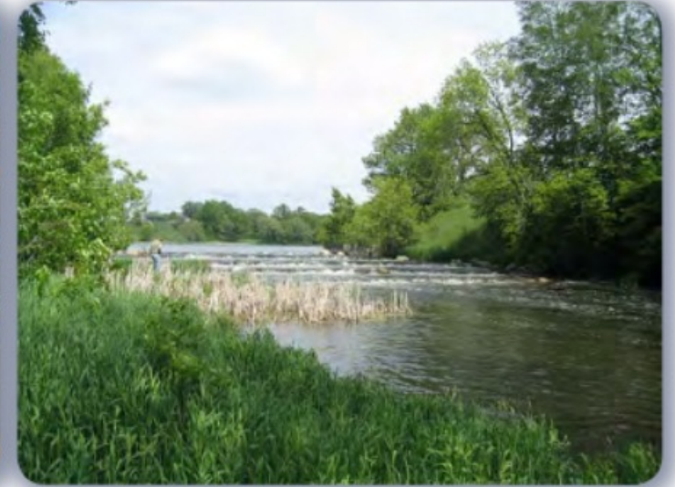
Upstream view of completed ramp
