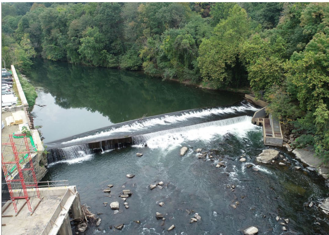
Photo 1. Aerial View of Dam 4 from Drone Showing Void on Left Side, Dated 9/25/2020
