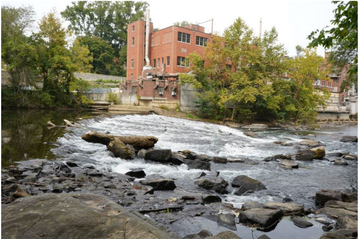
Figure 3. Dam 6 Viewed from the Right Bank
