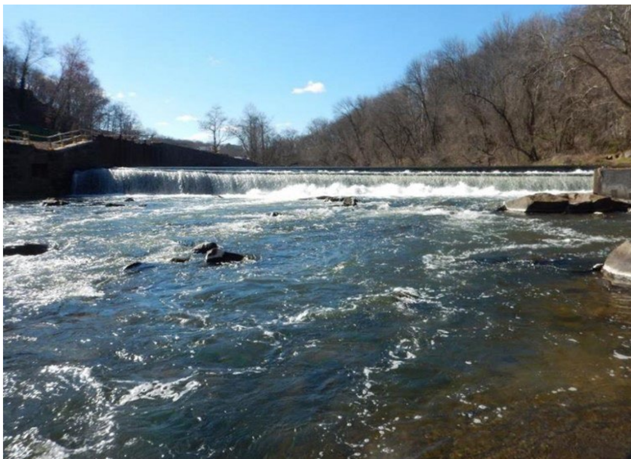
Figure 1. Dam 4 from River Right, Looking Upstream
