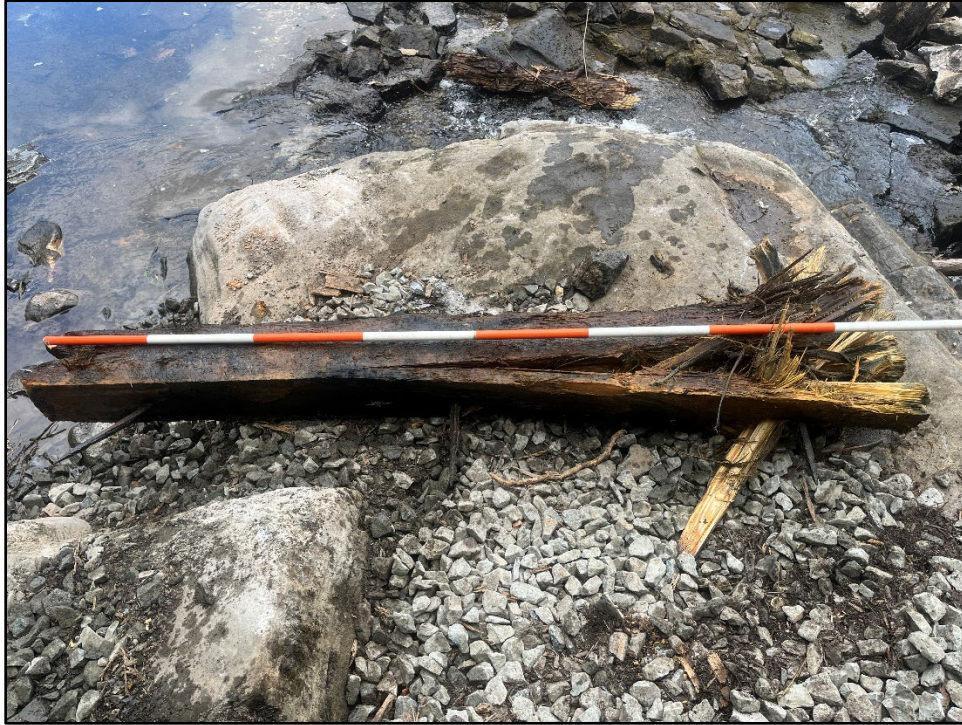
Plate 4.15: View of a large, square timber with ferrous metal spikes removed from the downstream portion of the dam during the initial breach. Photo view: N/A; Photographer: Jonathan E. Dernbach; Date: July 23, 2025.
