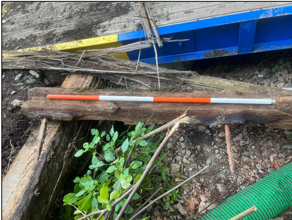
Plate 4.14: View of large, square timbers with ferrous metal spikes removed from the downstream portion of the dam during the initial breach.
