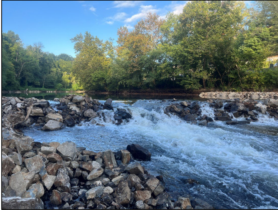
Plate 4.11: View of the loose boulders stacked in front of the downstream portion of the dam and the visibility conditions at approximately 50 percent breach progress. Photo view: West; Photographer: Jonathan E. Dernbach; Date: September 4, 2025.
