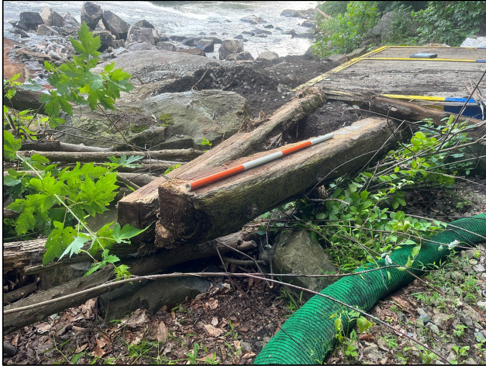
Plate 4.13: View of large, square timbers removed from the downstream portion of the dam during the initial breach.
