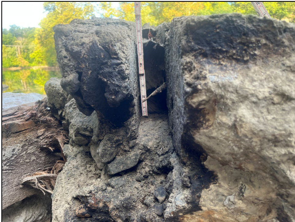
Plate 4.10: View of a milled board embedded upright in a removed portion of the concrete top of the dam.
