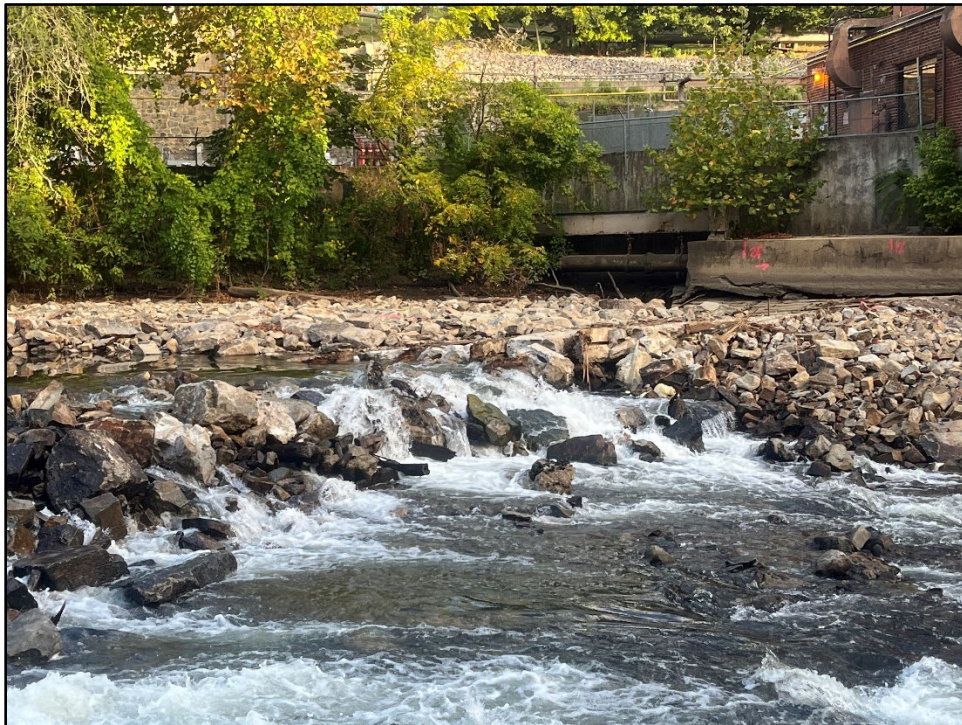
Plate 4.12: View of the cross section and front of the dam at approximately 50 percent breach. Photo view: Northwest; Photographer: Jonathan E. Dernbach; Date: August 2, 2025.
